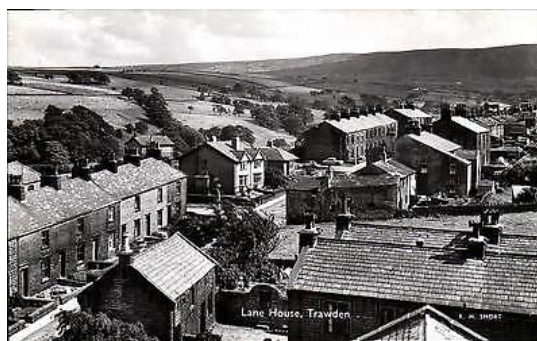
Lane House from the Church Tower
